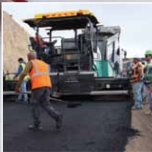
PAVING PROJECTS UNDERWAY
