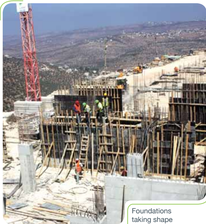
Workers pour concrete produced at Rawabi's on- site concrete batch plant
